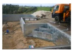
Detail of the Ingress Area (Note: Under the new Building Act 2004, we cannot refer to these features as "steps" as they do not comply with the Act for height. So we use "Ingress" and "Egress" - being Latin for "entry" and "exit" otherwise they cannot have a riser (vertical element) of more than 200mm. No good for sitting on in the pool water, would hardly dampen your bottom!
