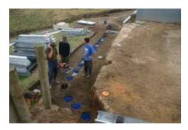
Finally all done! Buckets were used to stop the forecasted rain from filling the holes. Rebar steel hooked through the bucket handles was used to stop the buckets falling down the bore holes. It worked!
