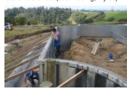
Peering over the abyss! Where the crew is standing will be infilled back up to 1.0m depth at that point. Due to the nature of the substrata. I suggested that some footpath mesh or Rebar used to stop localised subsidence of the concrete floor.
